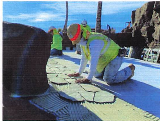
Mario Estrada carefully lays out stone decking near the pool
