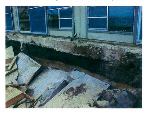
Unreinforced seawall fronting collapsed lanai area of Building F
