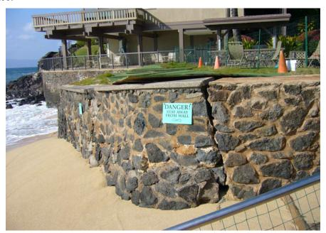
Figure 3. The wall seen in the photo above is shown with the recent damage caused by sinkholes in this February 2012 photo by Engledow. Signs, fencing and plywood covering sinkholes keep people out of the area.
