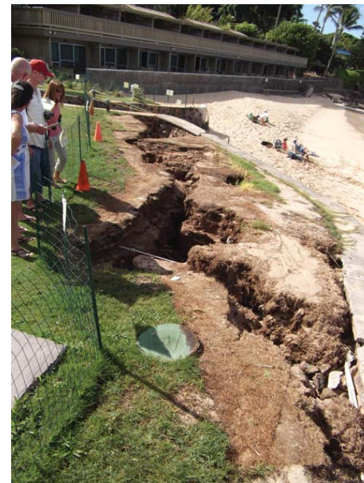
Photo 29: Sink holes behind seawall (10/10/2011).
