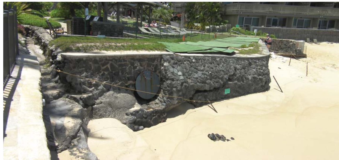
Photo 28: Existing seawall at 36-inch drainage outfall. Outfall will be relocated approximately 3-feet inland. Green plywood covers sink holes behind seawall.
