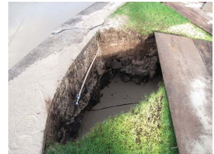
Photo 30: Typical sink hole behind seawall (1/10/2011).
