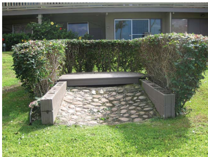
Photo 31: Top of 15-foot deep drywell (12/21/2011). 36-inch drain line from drywell to outfall at seawall will be replaced.
