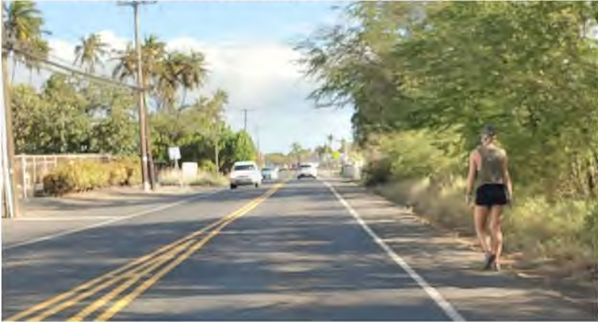
No Curbs, Gutters, or Drainage along SKR near Kauhaa St.:
