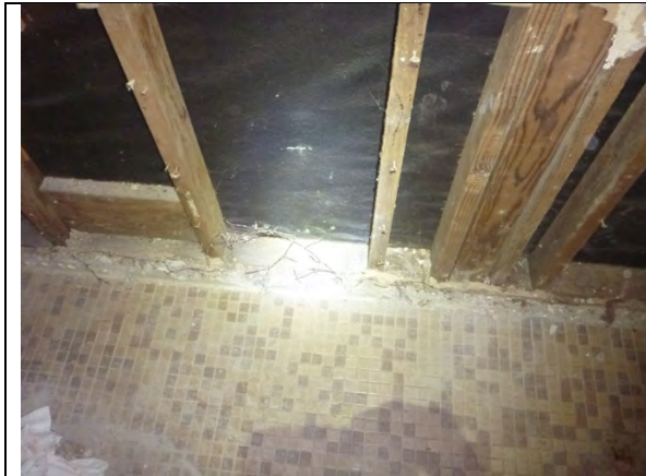
RC1CD.1: At various locations, sole plate anchor rods are installed at more than 32 inches on-center or missing.
