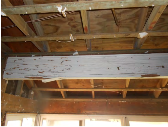
PBRD.1: Beam termite damage.
