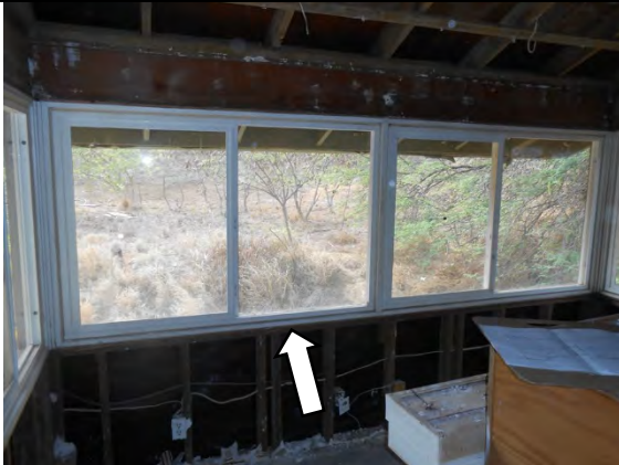
PC2CD.2: Wide opening with single sill plate.
