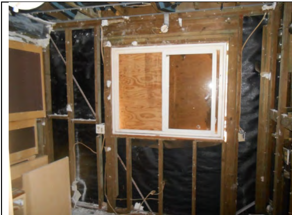
PC1CD.1: Missing opening king post.
