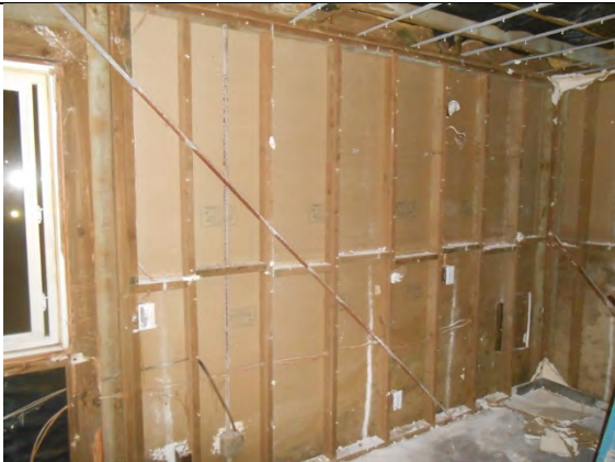
PB1D.6: Rusting steel wall braces.
