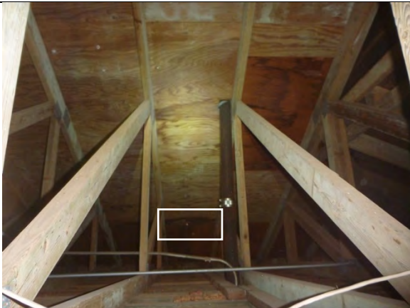
RCRD.2: Region of damaged plywood sheathing.
