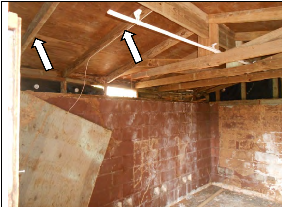
PTESB7: Damaged trusses. Missing truss framing.
