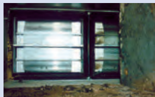
Photo 4C: Moldy air duct
