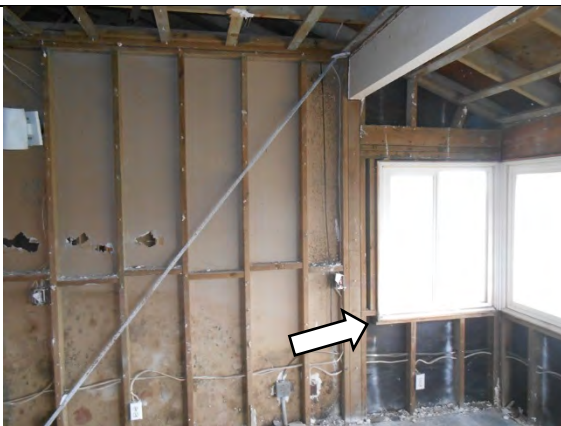
PC2CD. 1: Missing opening king post.
