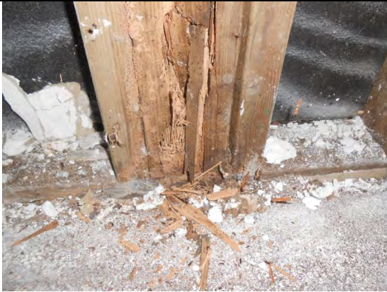
PC1D.4: Post termite damage.
