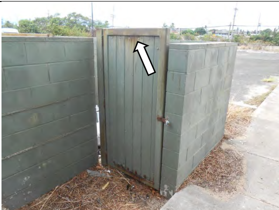
PTESB3: Rusting trash enclosure door.
