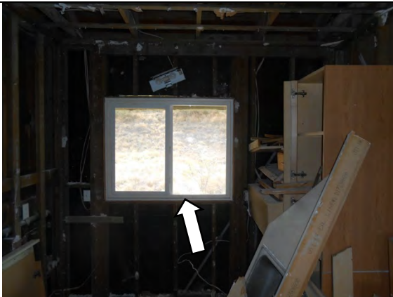
PC2CD.3: Missing opening sill plate.
