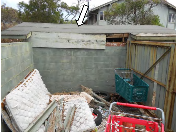
PTESB4: Damaged storage building roof.
