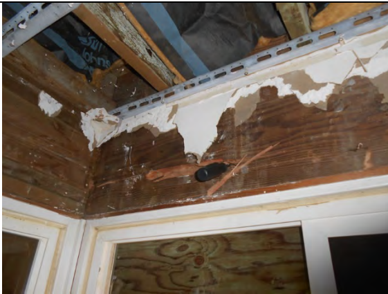
PB1D.5: Beam termite damage.
