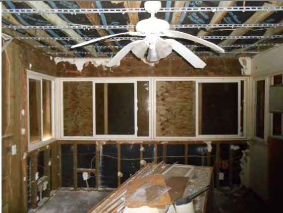
PB1CD.2: Wide opening with single sill plate.
