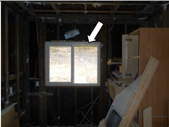
PC2CD.4: Missing opening header.
