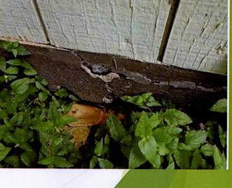
Exterior, Façade & Curtainwall: Rotted, <u>termite damage</u>, moisture damage
