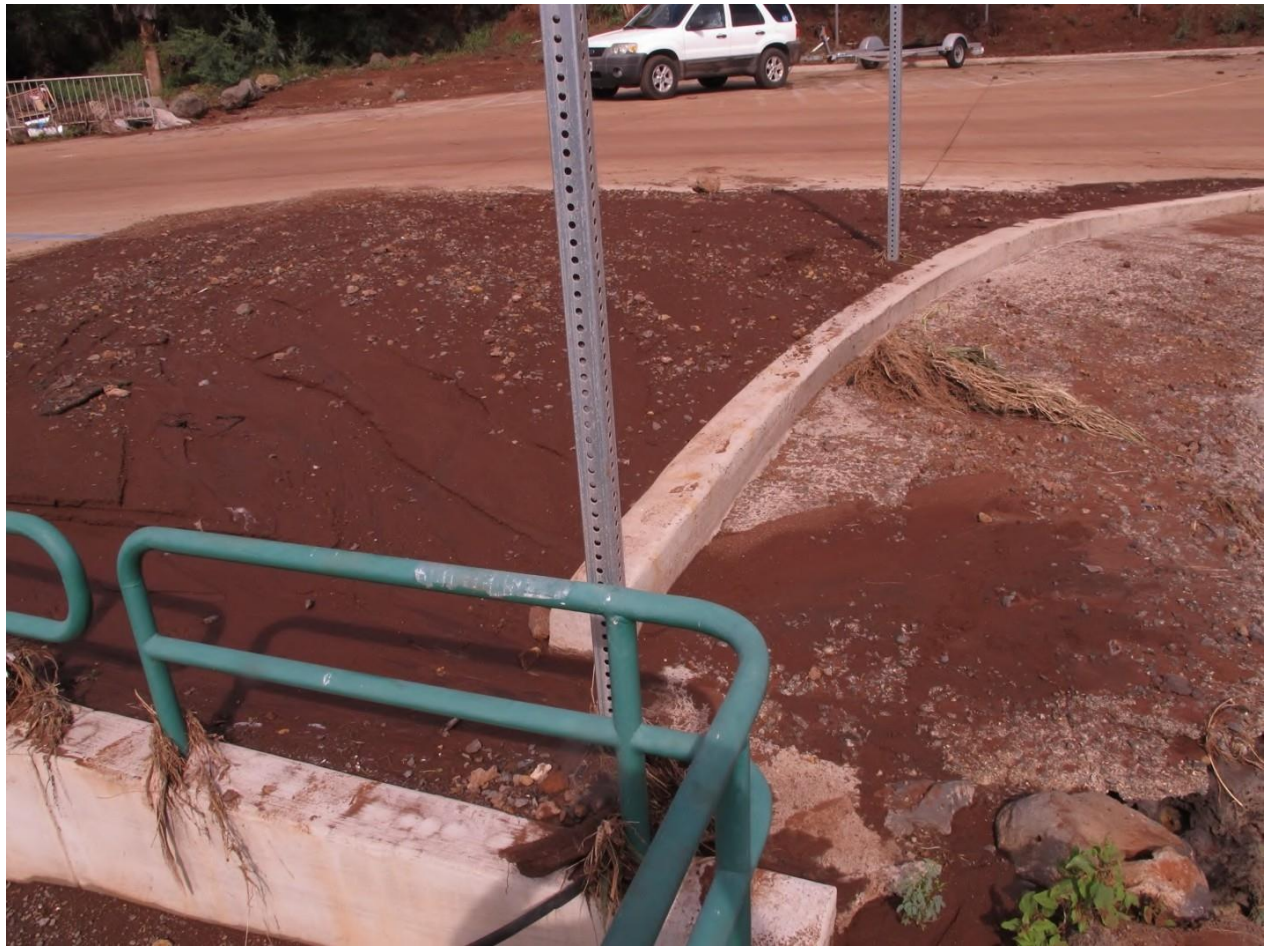
Figure 4 Sediment accumulation from culvert overflows onto parking lot near the boat ramp
