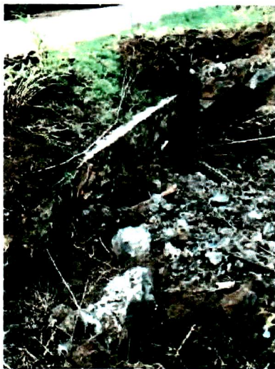
This is the upstream culvert which nearly complete obstructed on the opposite side of the road.
