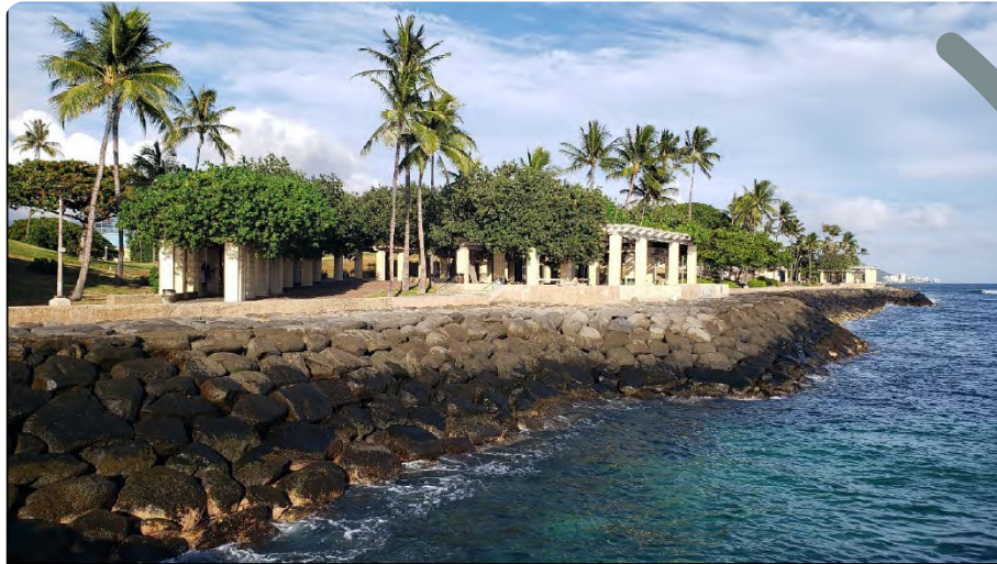
Figure 2-21: Rock Revetment at Kaka'ako Waterfront Park, Honolulu, O'ahu, Hawai'i
