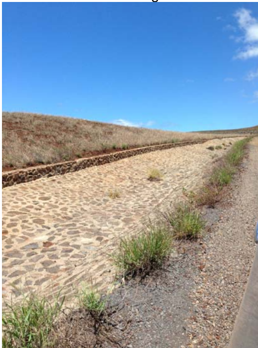
Photo 4: Landfill Drainage Swale
