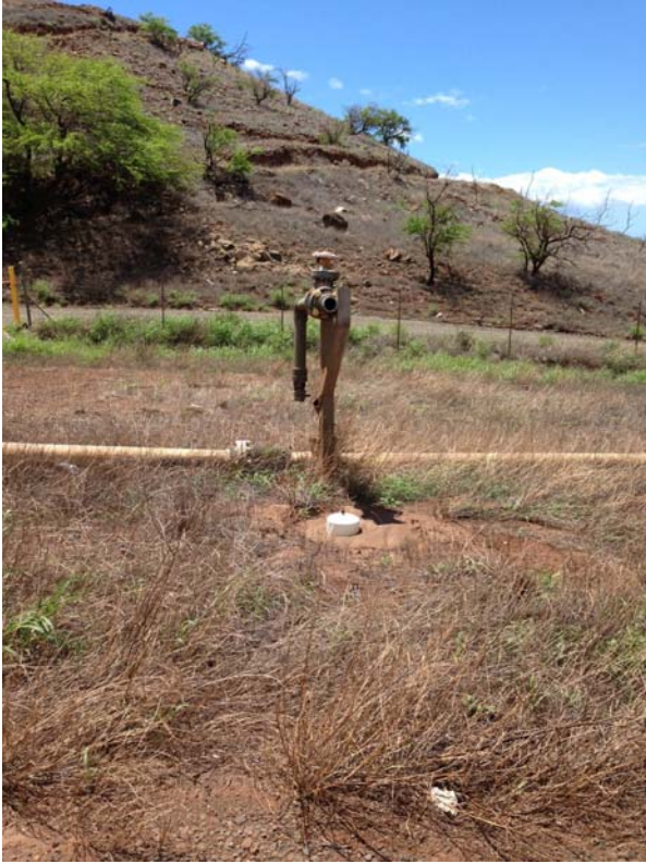
Photo 1: Landfill Gas System Port
