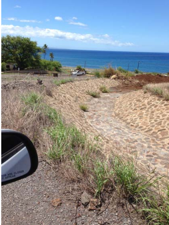
Photo 3: Landfill Drainage Swale
