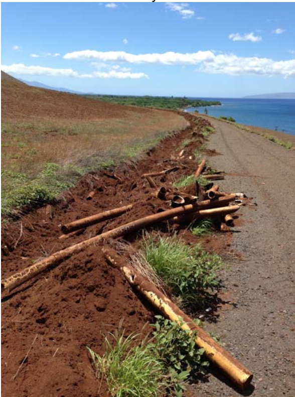
Photo 2: Excavated Gas Collection System
