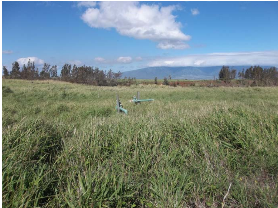
Photo C-6: Landfill Gas Trench Completions with Throttling Valve and Monitoring Port
