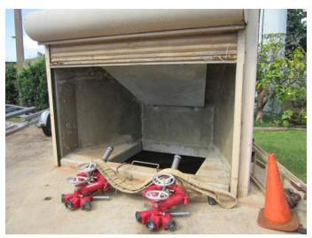
MFD Recirculating Hose Pump Test Pit
