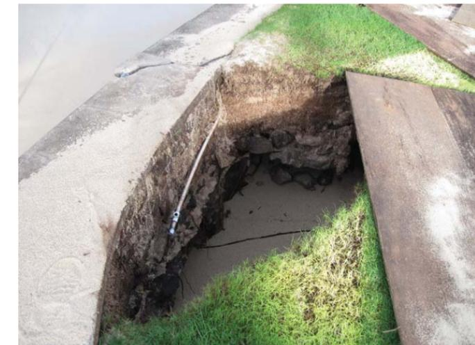
Photo 30: Typical sink hole behind seawall (1/10/2011).
