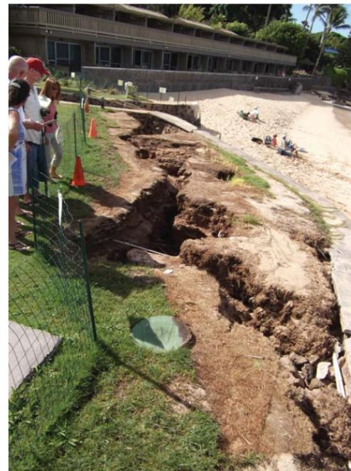
Photo 29: Sink holes behind seawall (10/10/2011).
