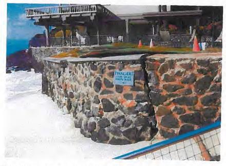
Figure 3. The wall seen in the photo above is shown with the recent damage caused by sinkholes in this February 2012 photo by Engledow. Signs, fencing and plywood covering sinkholes keep people out of the area.
