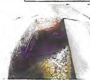
Photo 30: Typical sink hole behind seawall (1/10/2011).
