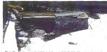
Photo 28: Existing seawall at 38-inch drainage outfall. Outfall wil be relocated approxi-mately 3-feet intend. Green plywood covers sink holes behind seawall.
