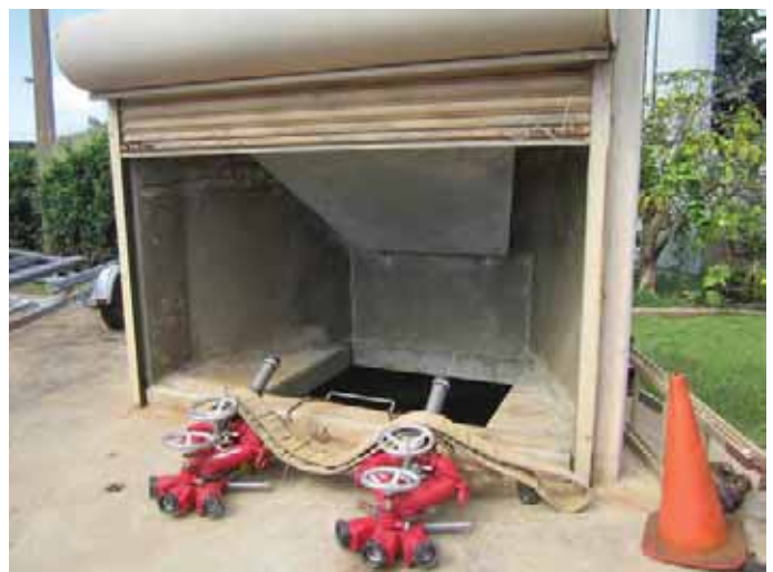
MFD Recirculating Hose Pump Test Pit
