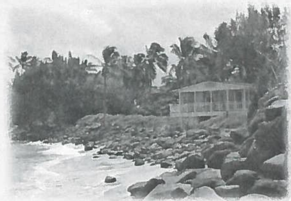
Figure 5. Revetments sloping walls made of large interlocking boulders - are less reflective to incoming wave energy than geotextile sandbags due to the spaces between the rocks. (Photo: Z. Norcross-Nu'u)
