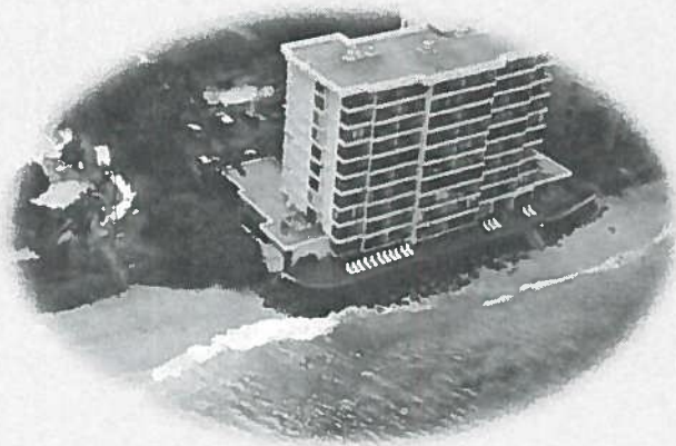
Figure 3. Shoreline armoring has led to the loss of the beach fronting this West Maui building. (Photo: C. Fletcher)
