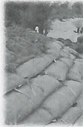
Figure 4. Geotextile sandbags have commonly been used for emergency shore protection on Maui. (Photo: Z. Norcross-Nu'u)
