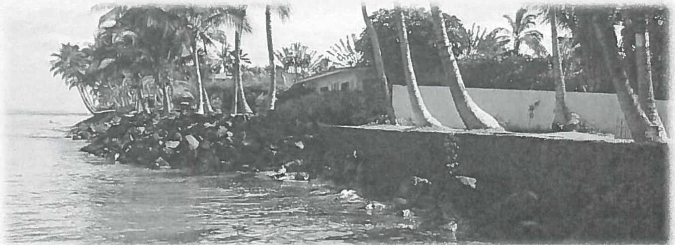
Figure e. A seawall (foreground) and revetment (background), built to protect private residences, have led to complete beach loss on this Kihei, Maui shoreline. (Photo: Zoe Norcross-Nu'u)
