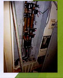
Main service conductors and all electrical branch wiring was cut at the main service panel entrance. Need electrical contractor to evaluate and repair electrical service to each building.
