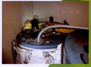
All water hearing appliances were terminated with supply and service plumbing cut and electrical connections removed. Recommend having a licensed pumber evaluate and install commercial grade gas on demand hot water hearing systems for each floor of each building
