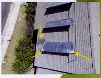
Plumbing: Non-standard repairs, <u>water heating devices terminated with</u> <u>supply cut and electrical connections removed</u>, solar panels damaged & leaking, fixtures in poor condition
