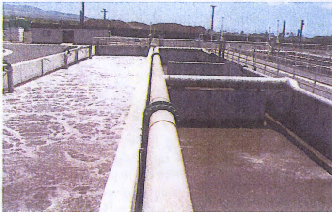
Figure 3: Kihei WWRF Flexible Aeration Basin
