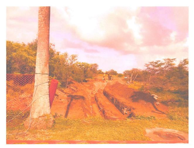
I was told before this project started that there would be 2 waterlines, one 12 inches in diameter and one 8 inches in diameter. They would be in about a 4 feet width configuration with 1 foot on either side. So I asked about 6a 6 foot wide trendh and how deep? The answer was 6 feet.
