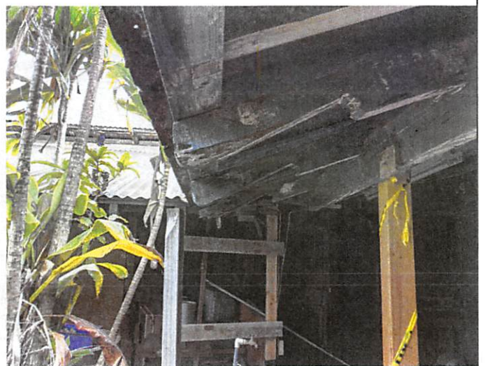
Stables, rounded rafters, birds mouth cuts. Structural damage stabilized
