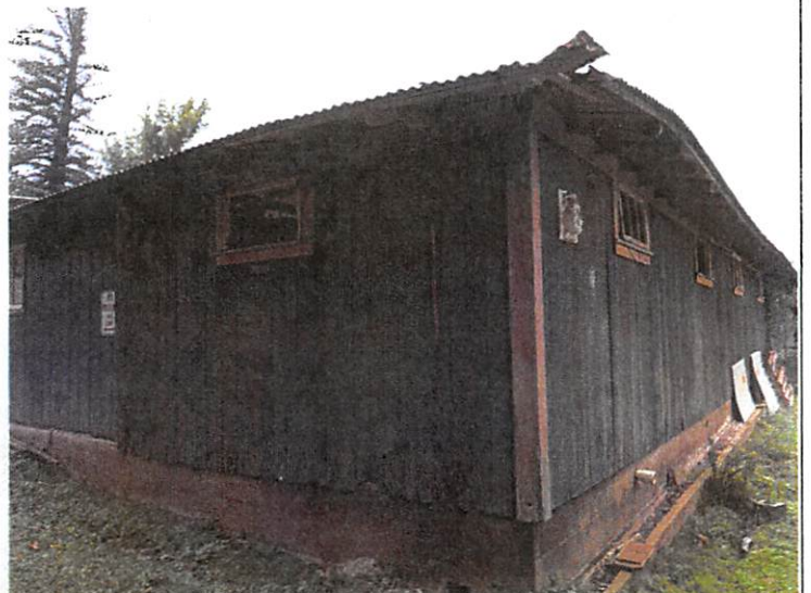
Stables, northeast corner. Erosion of siding and partial roof failure
