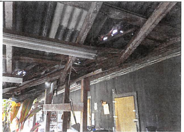
Stables, collapse of roof hip due to compromised wood framing
