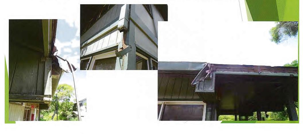
Roofing: Moisture intrusion, missing shingles, gutters damaged/broken/missing
