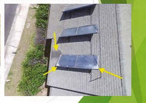
Plumbing: Non-standard repairs, <u>water heating devices terminated with</u> <u>supply cut and electrical connections removed</u>, solar panels damaged & leaking, fixtures in poor condition
