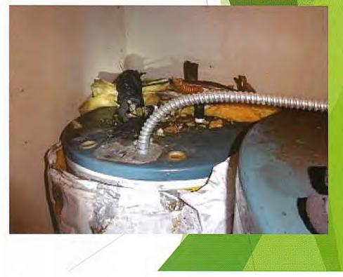
Plumbing: Non-standard repairs, water heating devices terminated with supply cut and electrical connections removed, solar panels damaged & leaking, <u>fixtures</u> in poor condition
