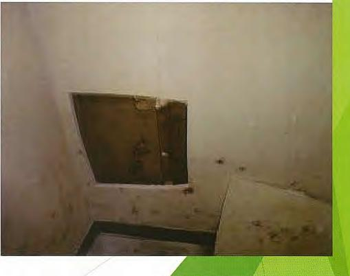
Interior Spaces: Moisture intrusion, mold growth and termite damage
