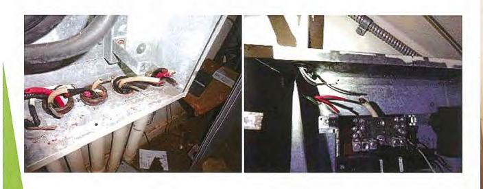
Electrical: Buildings B & C main service conductors and all branch wiring cut at main service panel, circuit breakers removed, missing junction boxes, <a href="mailto:improper repairs">improper repairs</a>
