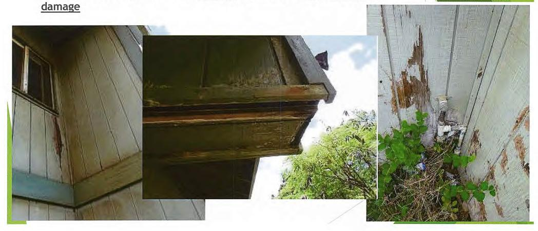
Fenestration (Exterior Doors/Windows): Termite, moisture damage, corroded, damaged & most inoperable
