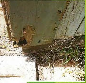
Exterior, Façade & Curtainwall: <u>Rotted</u>, termite damage, <u>moisture</u>
