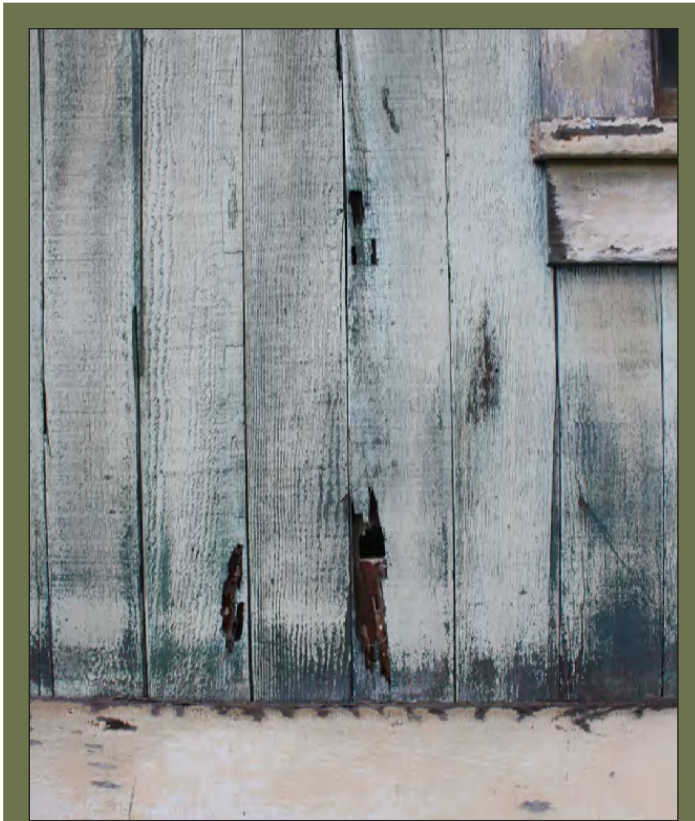
Pictured above is original tongue and groove siding. Repair original siding when possible instead of replacing or covering it.
