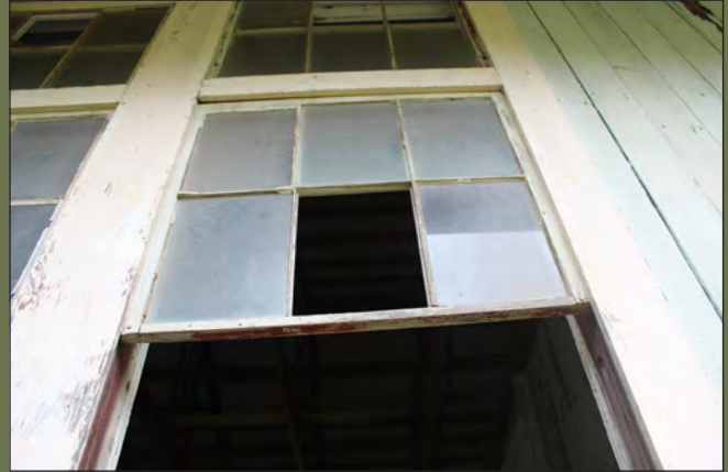
A missing piece of glass does not mean the whole window needs to be replaced -- just replace that one missing piece.
