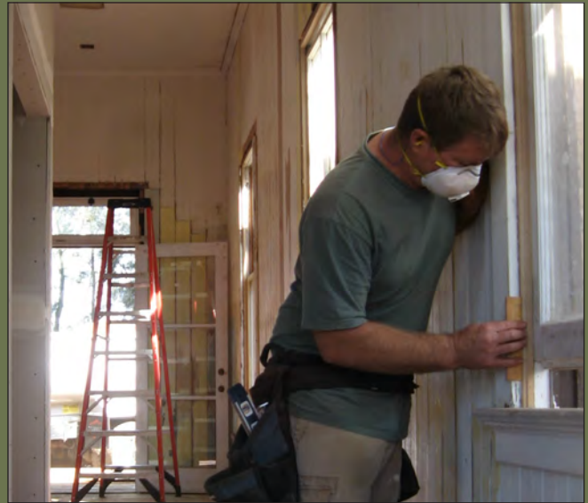
Repair original windows when possible instead of replacing them. Photo: Stanley Solamillo.
