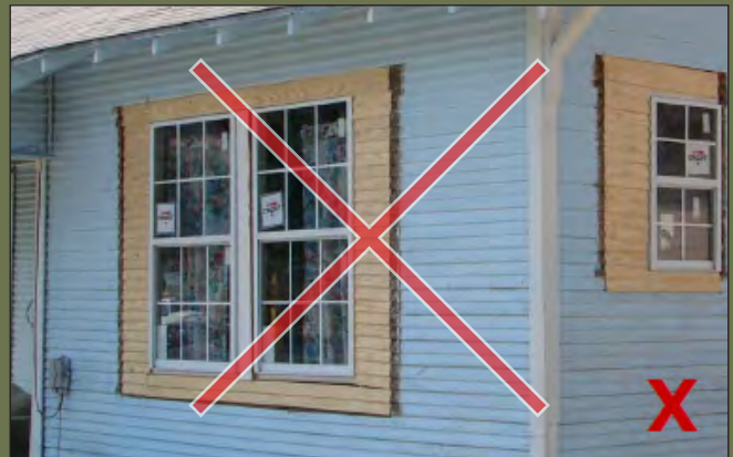
Do not change the shape or size of original window openings or use fake divided lights when replacement is necessary. Photo: sarehabberclub.com.
