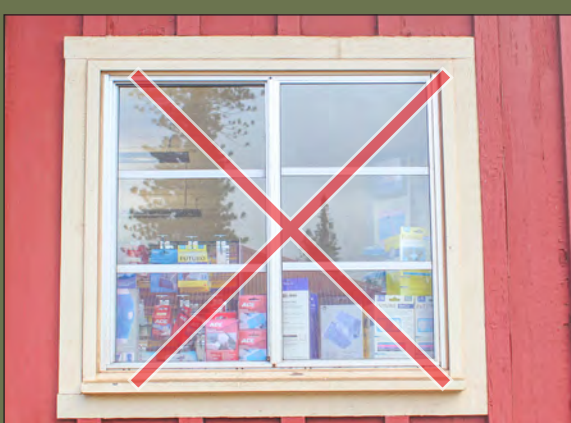
This facade's original windows and window components, including the trim, have been removed. The replacement windows are also a poor match for the originals.
