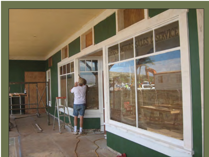
Instead of being replaced, these original storefront display windows were repaired in a way that preserved their historic character. Repair original windows when possible instead of replacing them. Photo: Stanley Solamillo.
