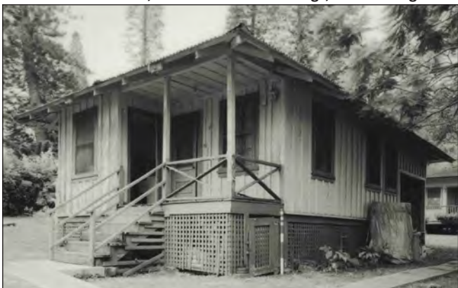
Porch Columns, Balustrades and Railings, and Skirting
