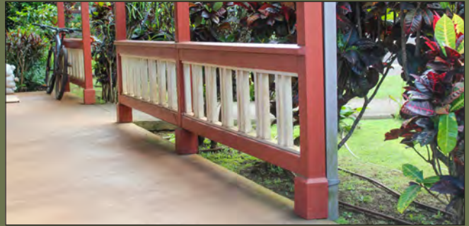
Preserve unique porch elements like these balustrades and columns.
