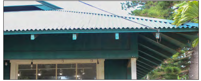
Deep eaves and exposed rafter tails are common roof features in Lānaʻi City.
