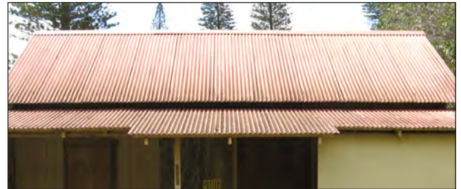
Corrugated metal is the most common roofing material in Lānaʻi City. Photo: Stanley Solamillo.
