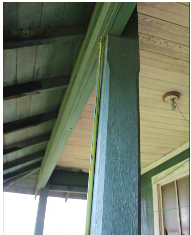
Exposed Rafter Tails, Porch Columns, and Ceiling
