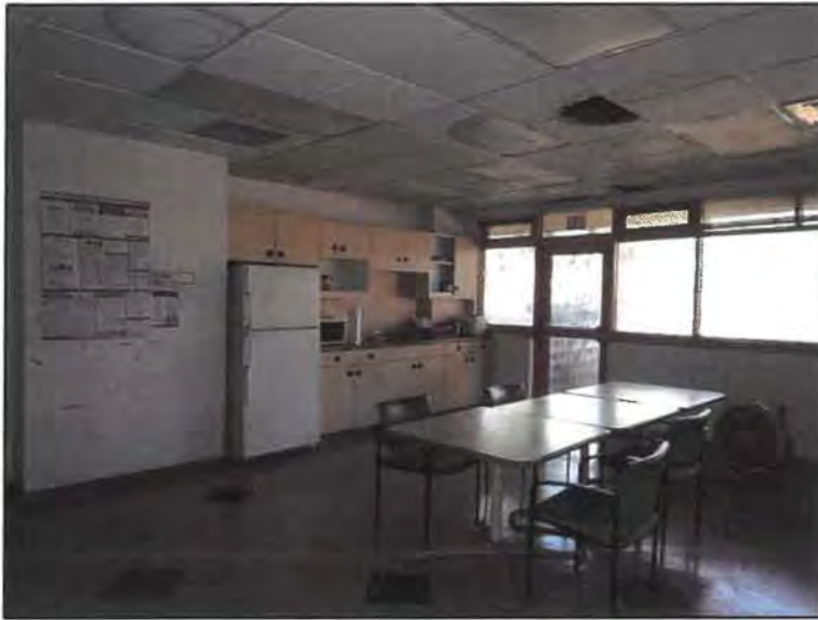
Interior view of break room in warehouse/office building. Note water damaged ceiling tiles are from previously leaking roof that was repaired in 2019.
