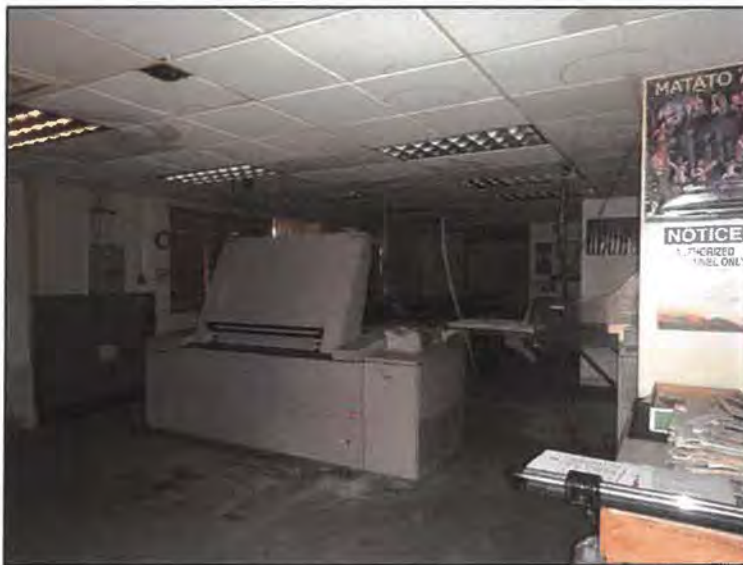
Interior view of workshop in warehouse/office building. Note water damaged ceiling tiles are from previously leaking roof that was repaired in 2019.
